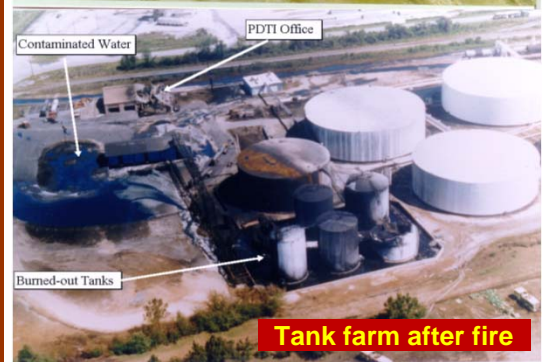
Tank farm fire
