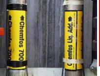
Similar labels on these pipes contributed to unloading the wrong material into a storage tank. A chemical reaction resulted, releasing a toxic gas which injured 6 people. See the April 2012 Beacon.
