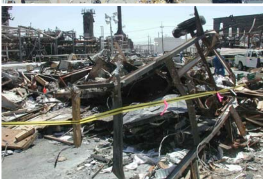
Damage to portable trailers from the March 2005 Texas City explosion
