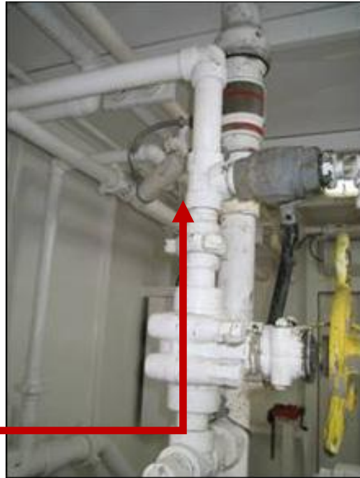
Above is a photo of the failed 250 psi valve. This valve was replaced with the appropriate 3000 psi valve
