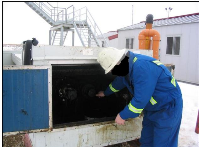
**Photo showing position of trucker when connecting and disconnecting load lines**
